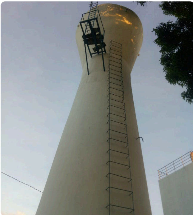
Rehabilitated water tower, Palma District (Phase 2 works)
