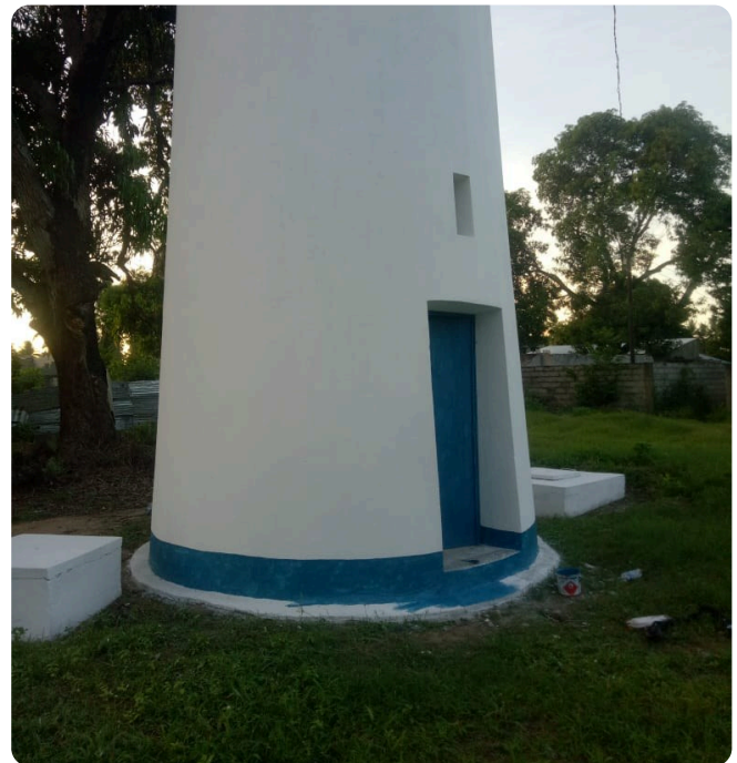
Tower base and access door after rehabilitation, Palma District (Phase 2 works)
