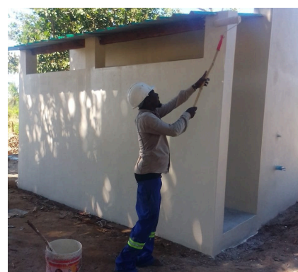
Gender-segregated toilet block at Muti Primary School, 2025
