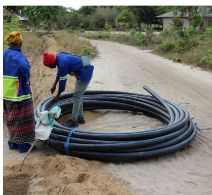
Laying the pipeline from the Quipuide tower to its fountains, 2025
