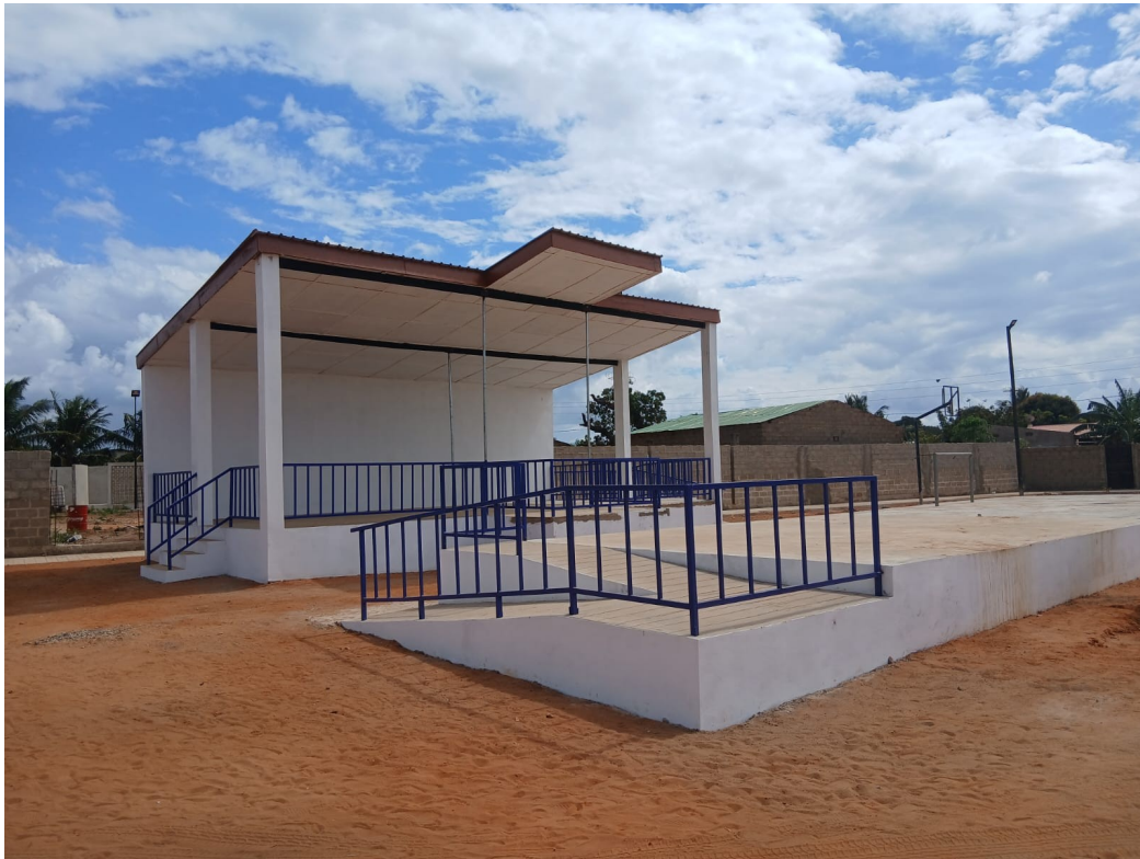
The covered community stage, with disability-accessible ramps and safety railings.
