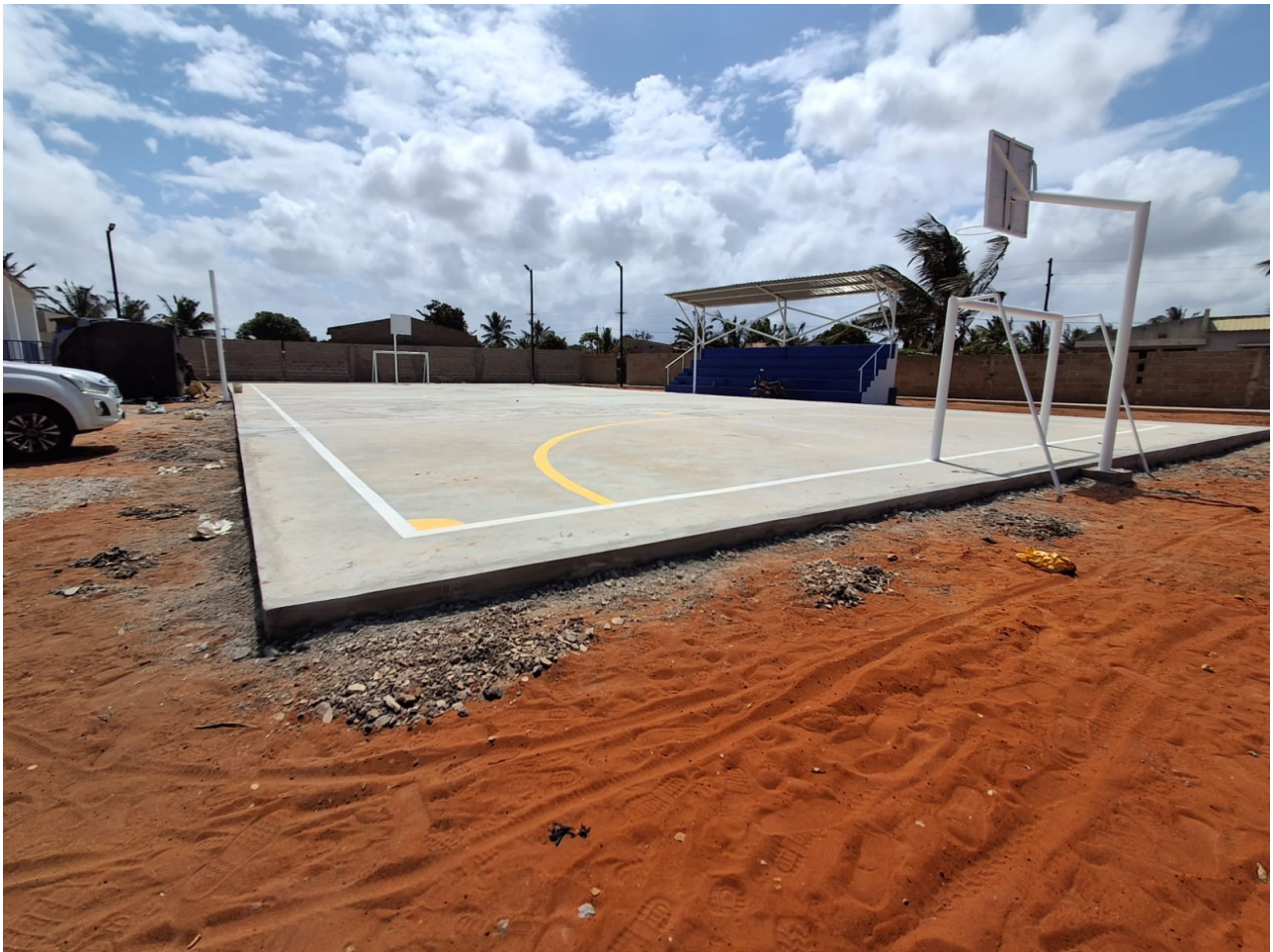
The completed multi-use court — basketball hoop, football goal and the covered grandstand beyond. Muxara, Pemba.
